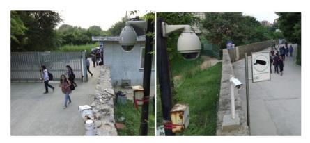
Figure: CCTV cameras can be installed for the purpose of surveillance. The images show CCTV cameras installed at the entrance of a premise to keep record of the visitors
