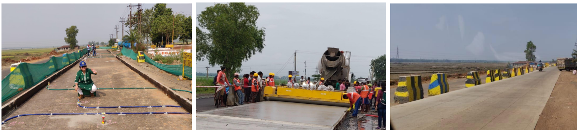
Figure 8.3: Instrumented 100m road with sensors for static and dynamic strain gauges, temperature sensors, pressure gauges and crack meters to be used for the Live Testbed.
